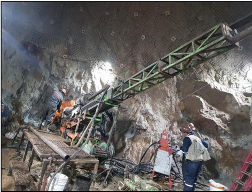
Figure 10.3 Drill Bay at Huayra Kasa Adit
